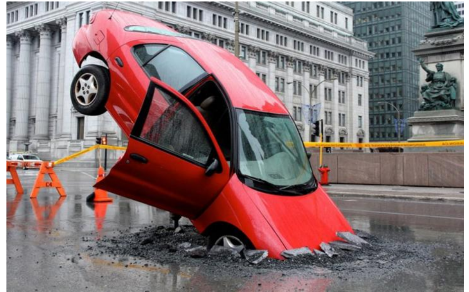
pothole in Montréal
